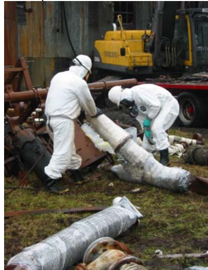
Asbestos Removal Operatives Clearing the site of material
